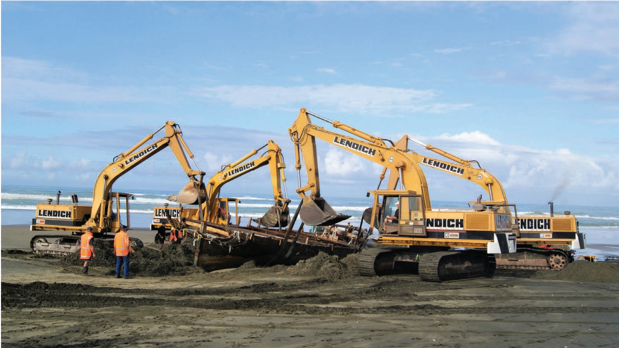
Fig. 3. Mechanical excavators lifting Daring from the beach at low tide, 12 December 2018. (K. Bennett, 2018).
