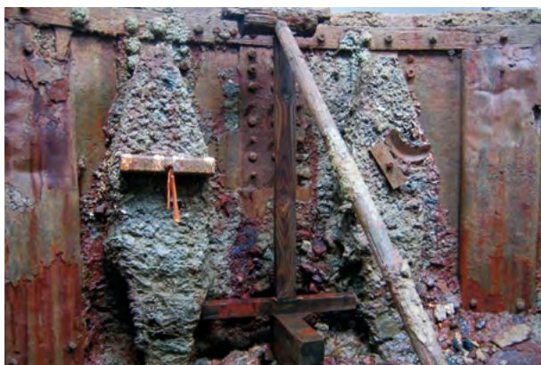
Figure 3: Internal walls of the Monitor turret showing the nut guards in position and the steaking patina of \text{FeO} . \text{OH} on areas cleared of concretion.
