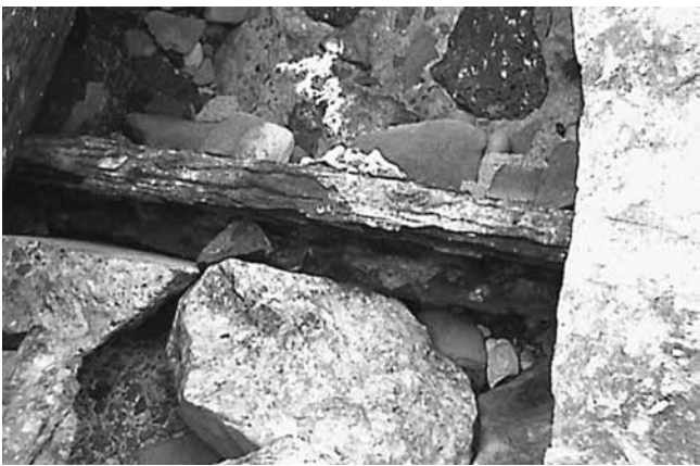
Figure 20. Steel rail lines c.1999. Slipway for SS Dumaresq , 1909.
