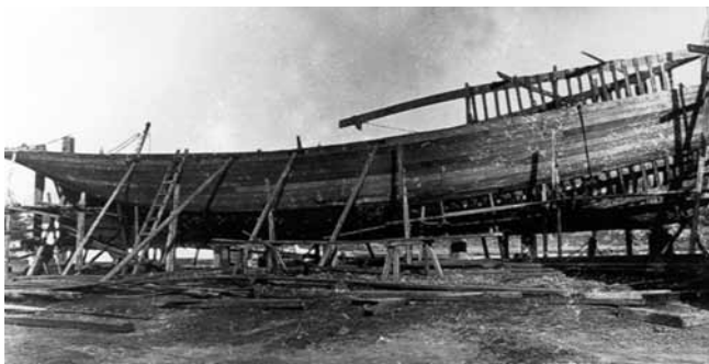
Figure 7. SS Dumaresq . Spotted gum planking being attached to the frames (Courtesy: Alfred Settree, 1995).
