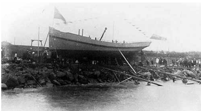
Figure 9. Completed hull of the Dumaresq prior to launching. Note the railway lines forming the slipway. The rails are unequal length and positioned at slightly different angles to turn the vessel to the right upon entering the water (Courtesy Mavis Settree, 1998).
