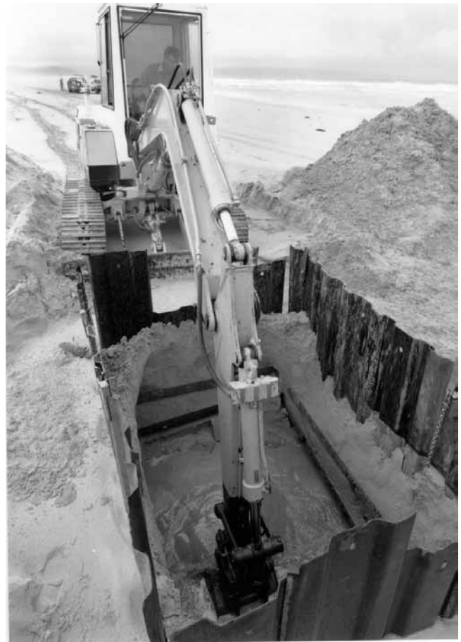
Figure 9. After the first metre, hydrated sand flowed into the hole. (Photo: S. Humphries)
