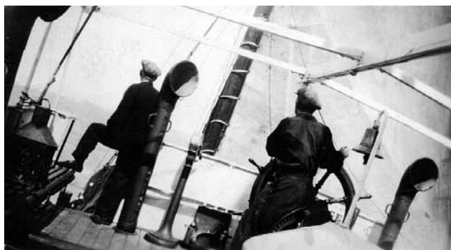
Figure 4. Visible in this photograph is a seat fitted along the inside of the handrailing, the belfry mounted on the skylight, and the timber frame on iron stanchions which supported the canvas awning. The binnacle cover has been removed and placed on deck next to the engine room telegraph. SAMM:8101 .
