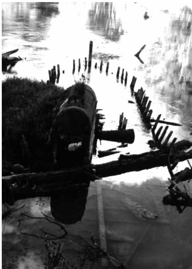
Figure 6. A multitubular boiler on the remains of the PS Banyula wreck site, NSW. Kenderdine, 1993.
