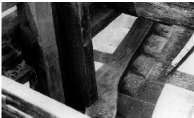
Figure 11. Evidence of the rotting effect on coconut wood lugs.
