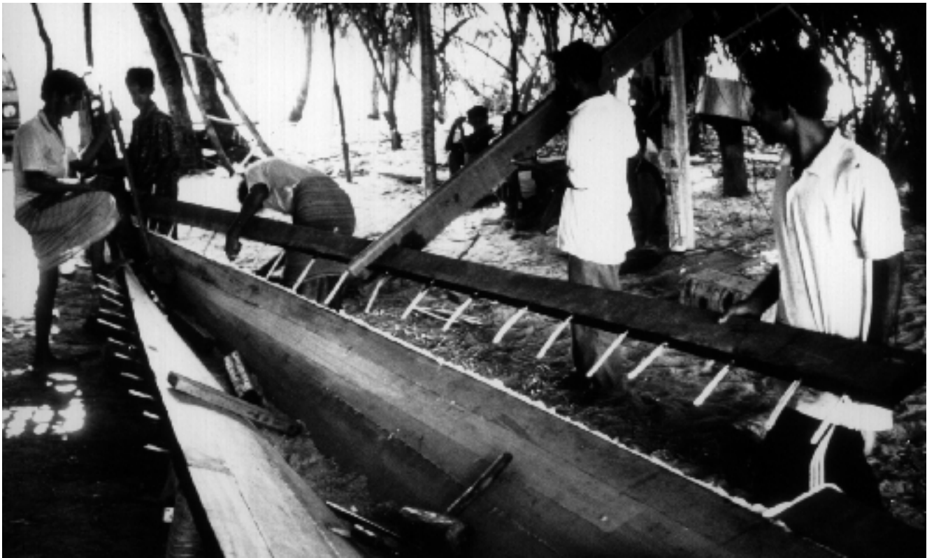
Figure 9. The new plank being fitted to the hull which has been prepared with cotton wool.
