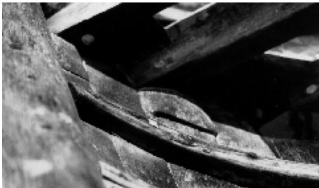
Figure 3. Lugs positioning the thwart beams.
