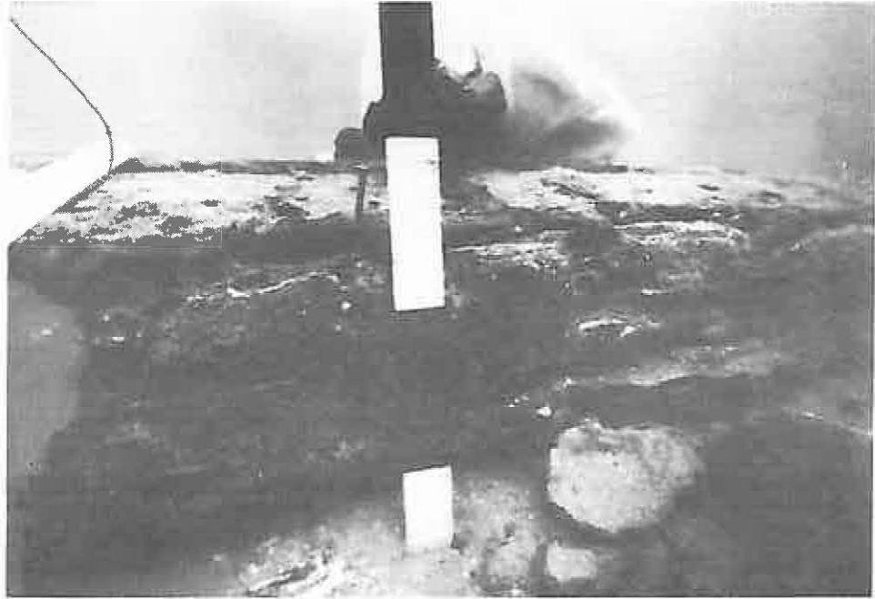
Figuer 10A. Planking at edge of site showing layers.
